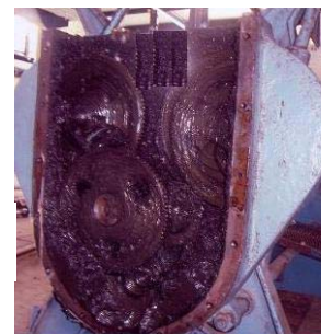
FIGURE2 Grease application in existing DR gin
